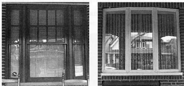
Left, preserve original windows. Right, an inappropriate window replacement.
