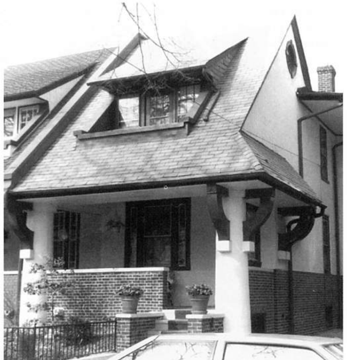
Bungalow – A product of California, the bungalow celebrated the organic relationship of man and nature. Typical features of this style include strong low-slung rooflines with dormers, massive columns, and a mix of materials, including stucco, stone and brick.
