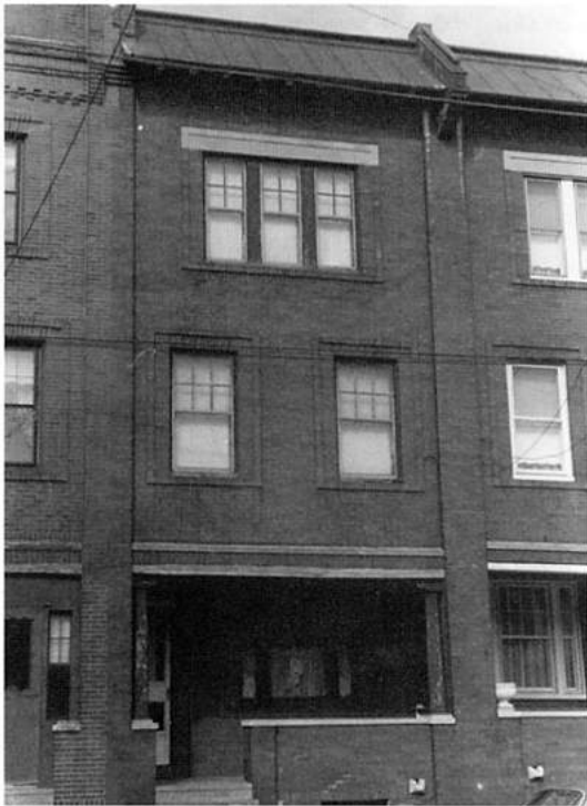
Arts and Crafts – Emerging from the British and American Arts and Crafts movement, this architectural style emphasized the tactile qualities of building materials and incorporated simple “honest” decoration, such as brick patterns, geometric designs and overhanging eaves.
