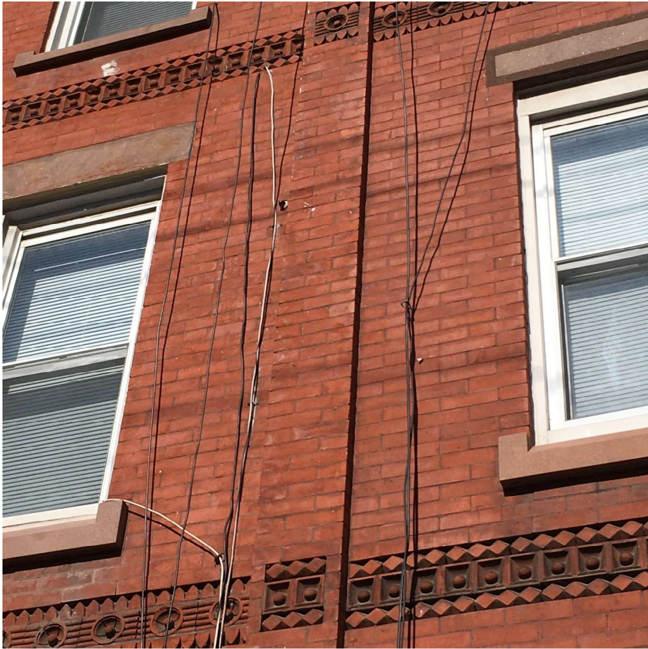
Figure 17. Brick courses on 3937 (right) and 3939 (left) Baltimore Avenue showing the delineation of floors. The decorative brick courses have been reversed from second floor to third floor.
