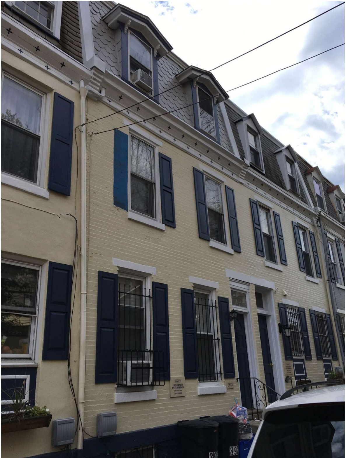
Figure 14. 3922 Delancey Street. This is a typical rowhouse with the original slate roof and the decorated cornice. The window sizes have not been changed although all the windows on this street have been replaced.
